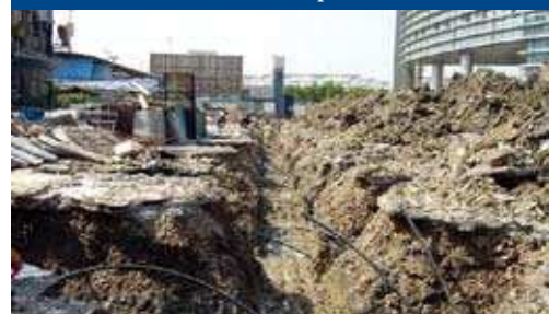
Pic. 4 | Geothermal Heat Pump Site Work
